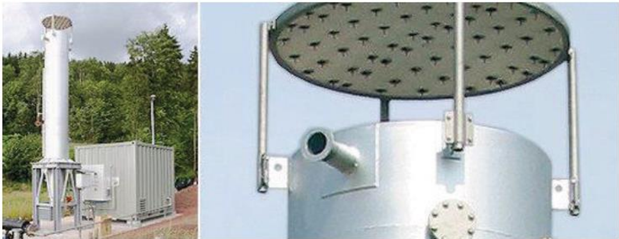
Figure 10-29: Gas venting station and high temperature gas flare
