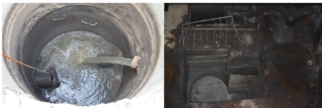
Figure 4-20: Main wastewater pumping station MWWPS-2, the town of Cupcini: Contact chamber. Receiving tank
