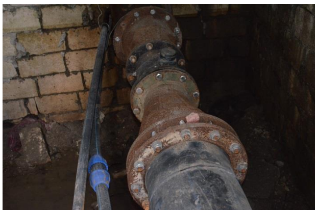
Figure 4-11: Manhole with water meter node for the town of Edinet
