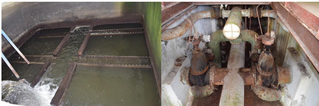
Figure 4-3: Water treatment plant. Open quick filter. The pipes of open quick filters
