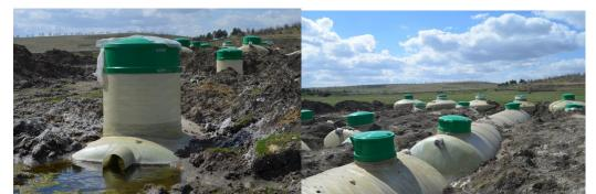
Figure 4-11: Traidenis container WWTP (Republic of Lithuania) under construction
