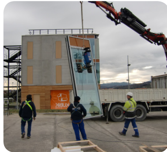
Demonstration Building KUBIC -TECNALIA
