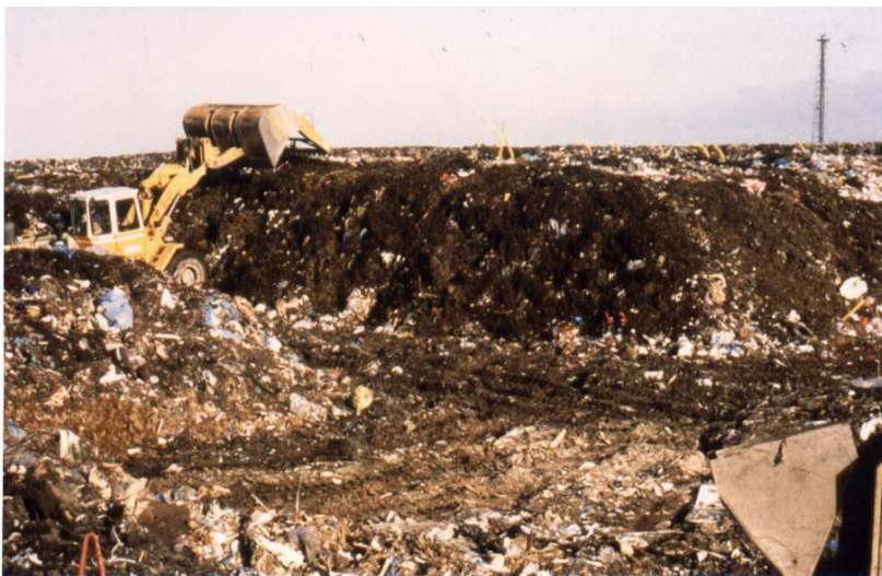
Figure 5-12: Chimney effect - set up of piles
